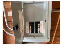
**84:** GENERAL: The subpanels were opened and the inspected circuitry was found to be installed and fused correctly.
