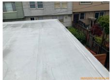
**67:** There is evidence of shallow ponding at the center of the roof. The presence of shallow ponds of water immediately after rains are not unusual, but regular maintenance of these areas is vital to avoid a buildup of rotting vegetation.
